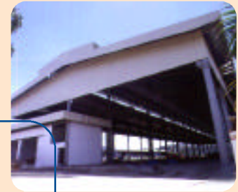
Construction of new factory building-in-progress
