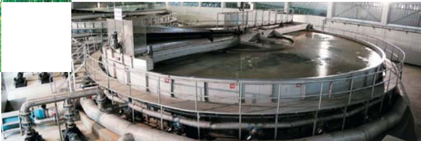
Pinang Water Ltd's, water treatment plant in Yichun
